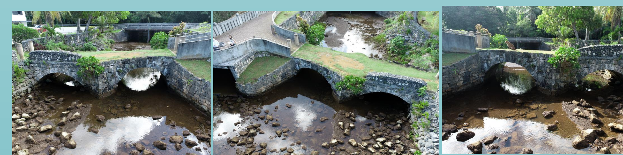
Taleyfac Bridge 2D drone image
