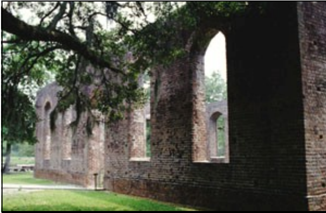
Surviving wall of St. Philip's Church in Brunswick Town dates back to 1754. The British burned the original structure to the ground during the American Revolution.
