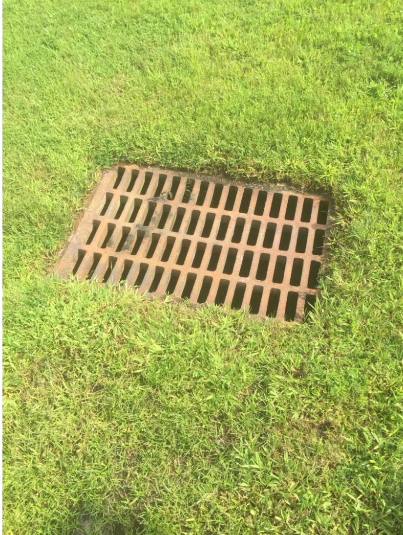
Figure 35. Photograph of grated manhole covers located in the yards of Cold Stream Cove and Summerall Oaks. The water which flows into these manholes travels to the pond via stormwater piped systems.
