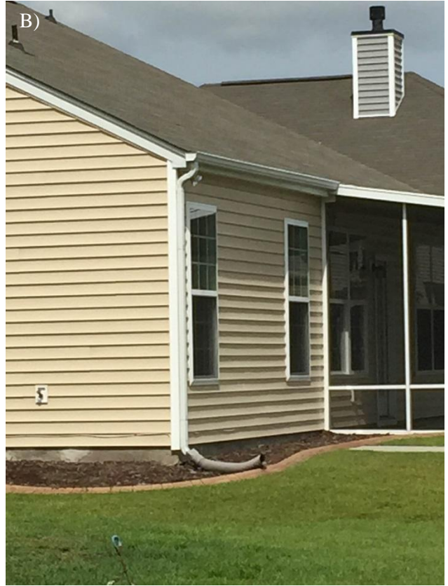
Figure 27. Photographs of the steep rooftops at Summerall Oaks (A) and the drainage pipes directing runoff towards the pond in the form of sheetflow across the yards surrounding the pond at Summerall Oaks (B). Similar drainage pipes are observed for the single condominium adjacent to the pond at Cold Stream Cove.
