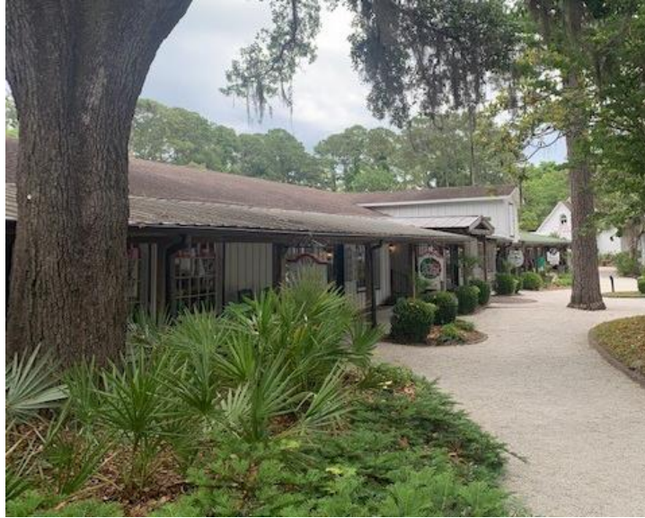
Figure 11: Angled view from the left side of the front of the original Hammock Factory. (2022)
