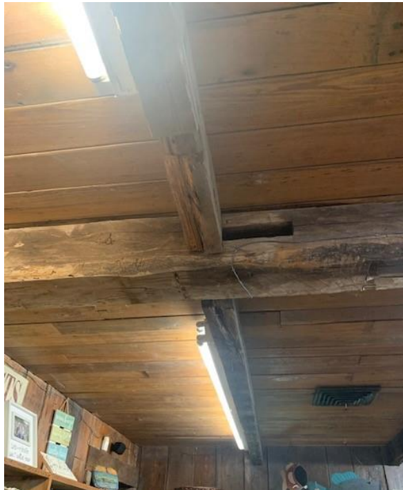
Figure 4: Hand-hewn beams from Maryville Planation. Interior of Original Hammock Shop. (2022)
